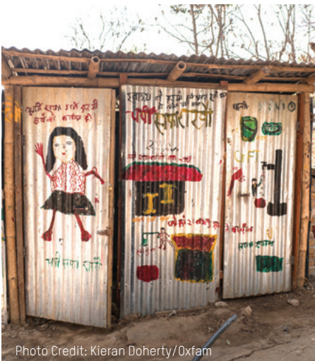
Oxfam installed Girls Toilets
