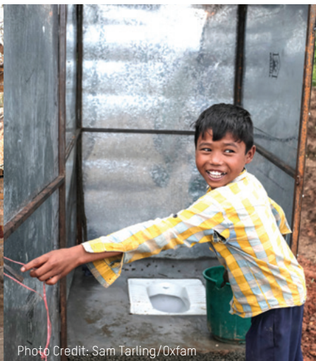
Oxfam installed toilet
