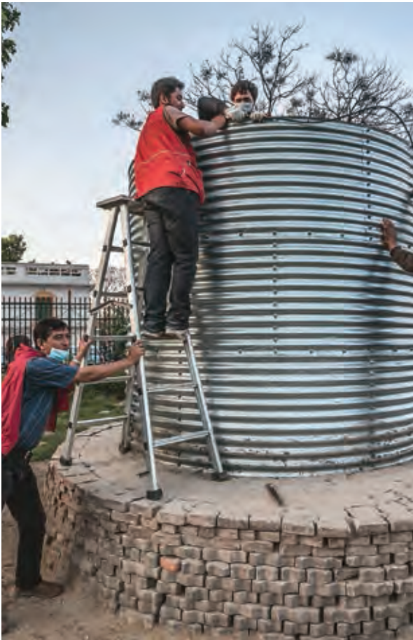
« A 11,000-litre water tank is being installed and 20 pit toilets constructed.
