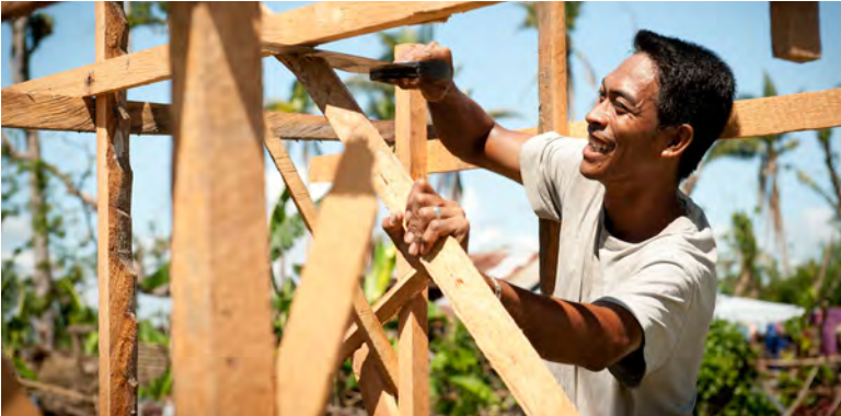
Larry Tondo, a carpenter and chainsaw operator in Oxfam's cash-for work programme, builds a sales kiosk from coconut lumber. Photo: Eleanor Farmer/Oxfam.
